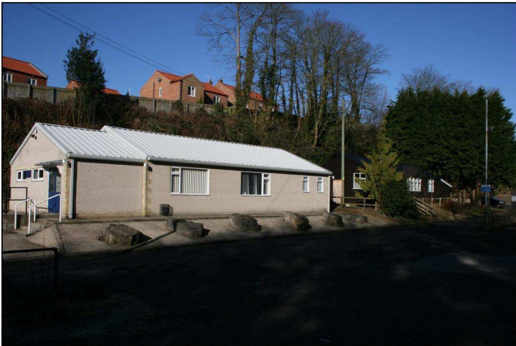
5 Band Hall viewed from development site
